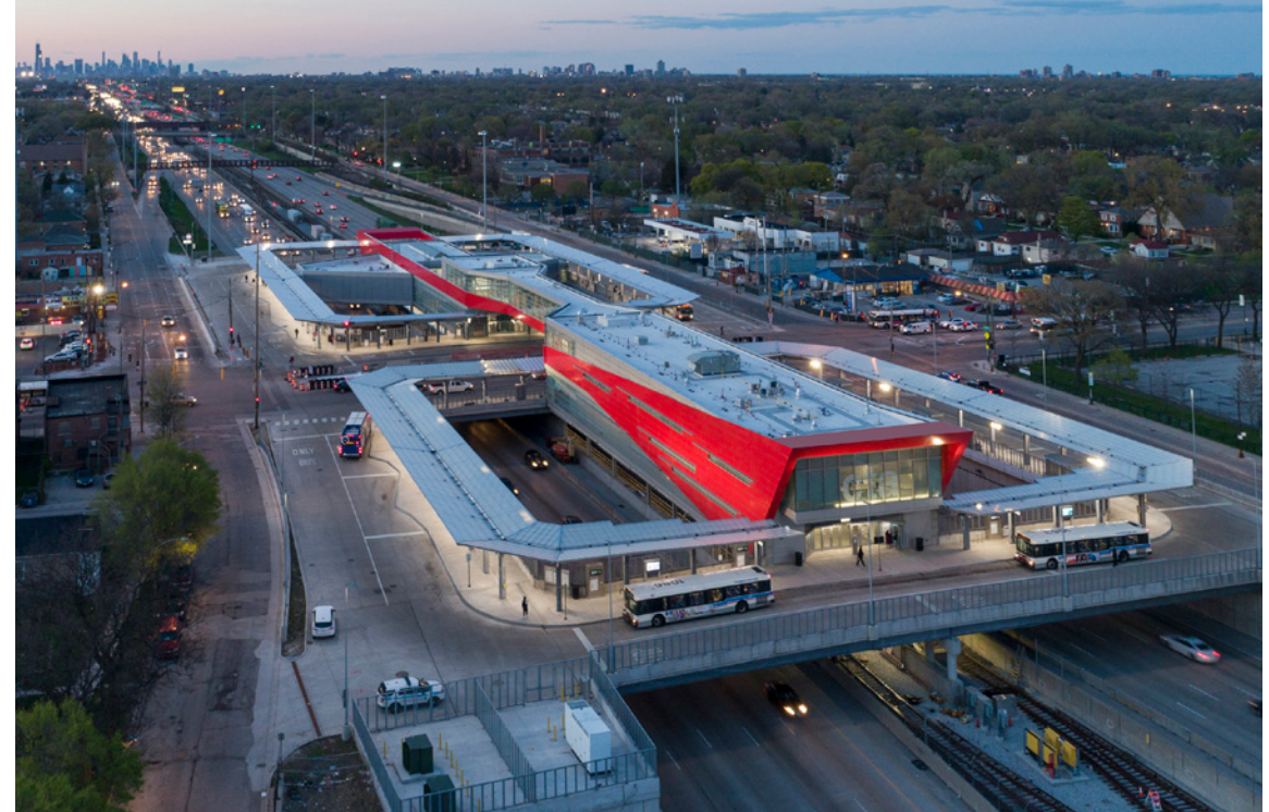
[Left] An aerial view of the 95th Street/Dan Ryan Intermodal Chicago Transit Authority station. Photo: James Steinkamp Photography
